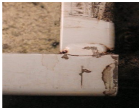
Figure 2. Pallet showing crack in weld.
