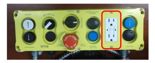
The GFCI will function; it will open both hot and neutral sides and the internal test button will trip the GFCI. However, the hot and neutral will be reversed on connections to the outlet and voltage may be present where none is expected. An external polarity tester may not trip the GFCI.
